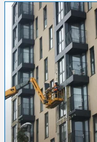
Cladding removal at Kennedy Gardens, Billingham
