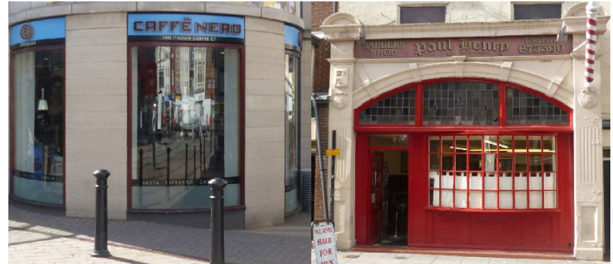
Above: Examples of both modern and traditional approaches to shop frontages
