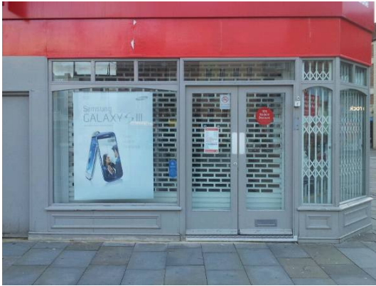
Above: Security grilles within the shop front
