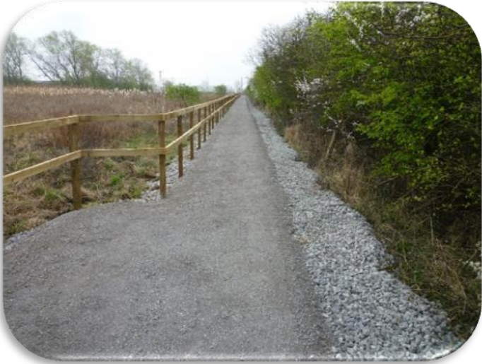
New Causeway (view towards Brine Pumping Station)
