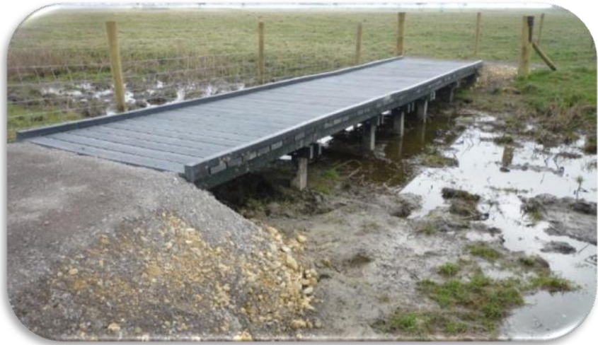
New boardwalk (north of A1185 roundabout)
