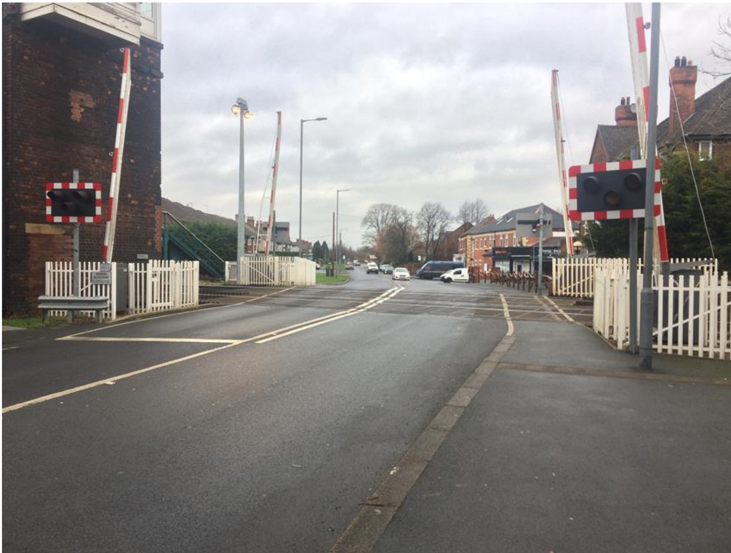
Station Road, Billingham
