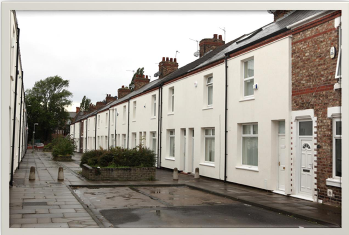
Housing improvement through External Wall Insulation in Stockton-on-Tees under the ECO programme
