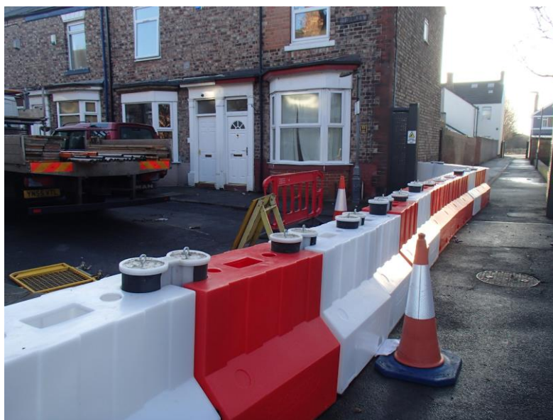
Stockton Council Flood Barriers at Bedford Street, Stockton
