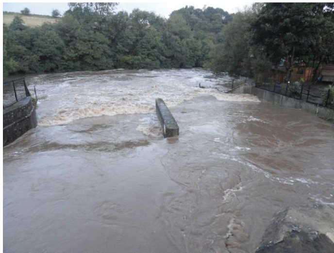
Leven Bridge – September 2012
