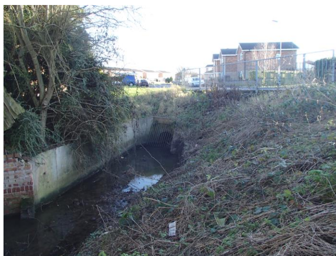
Surbiton Road – January 2015 (after work)
