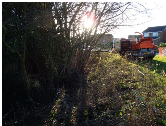
Surbiton Road – December 2014 (before work)
