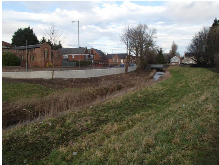
Bishopton Road – February 2015 (New flood wall)
