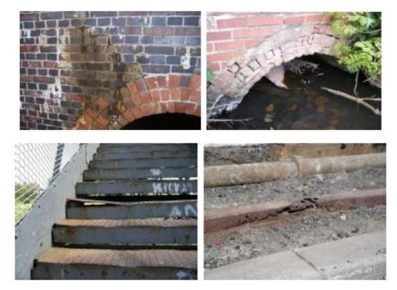
3.3 Members were informed that common problems included water and salt penetration, corrosion, loose bricks, cracks and flooding. It was subsequently important that gas pipes and other services were protected when carrying out maintenance work on structures.
