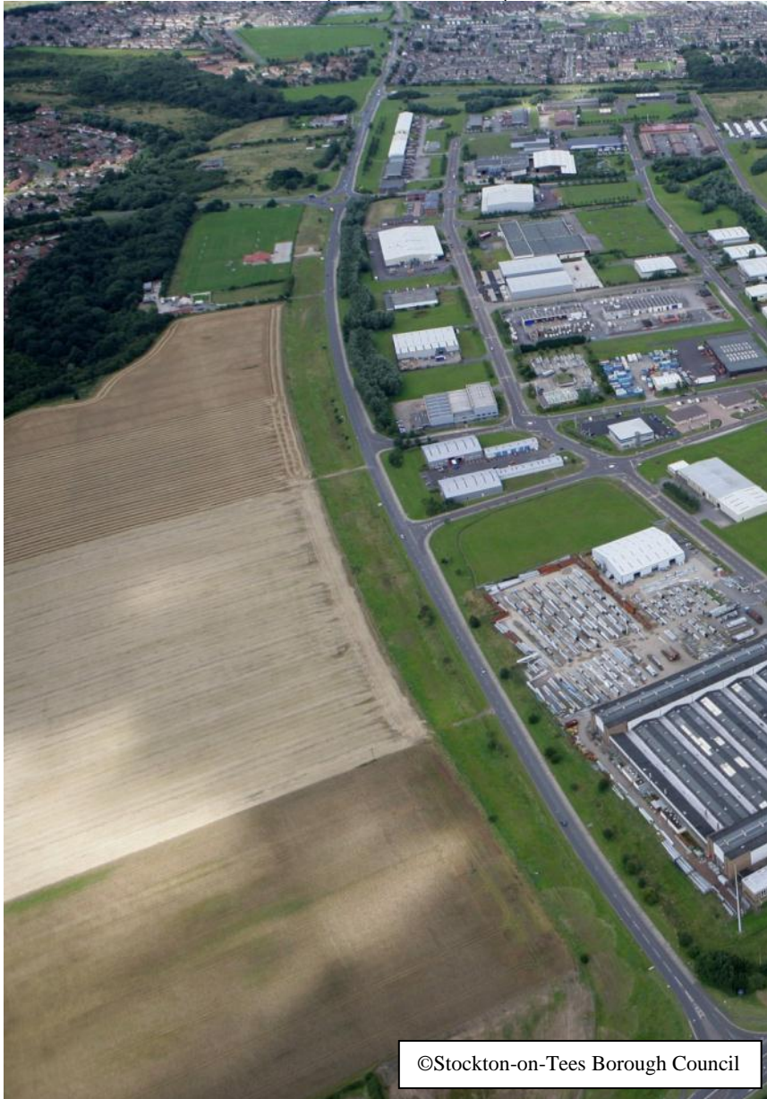
Areas 3 and 4 from Low Lane (northwards view)
