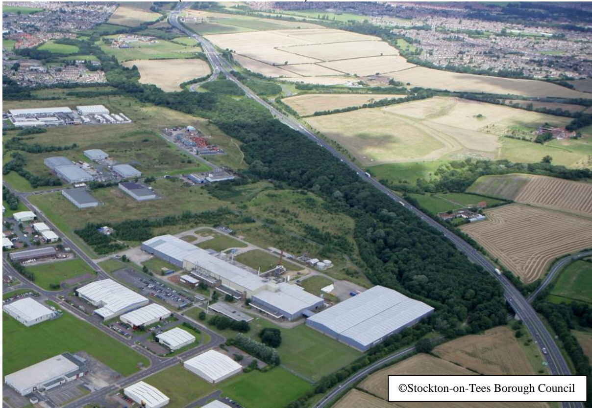
Areas 3 and 4 from Low Lane (north eastwards view)
