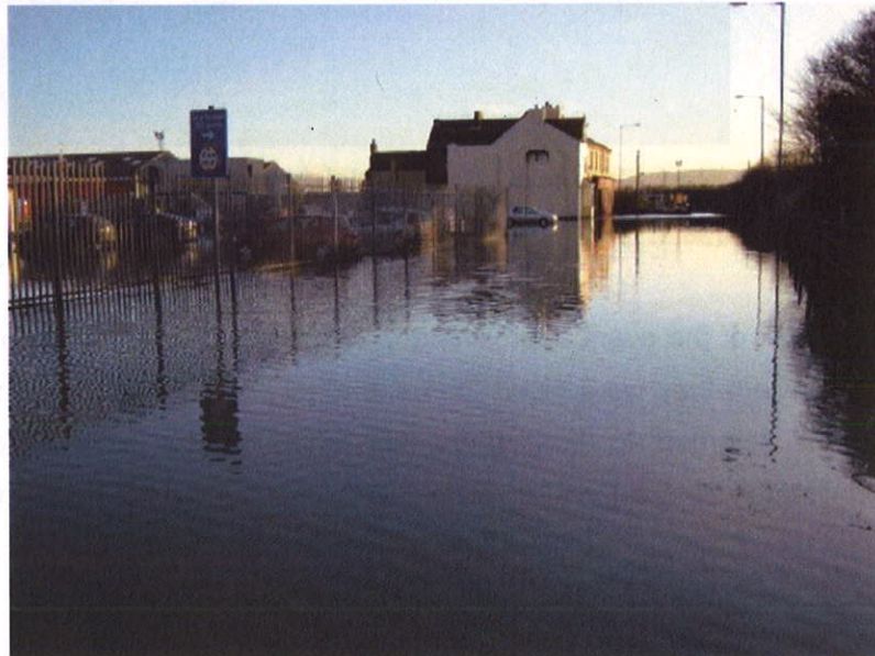
Port Clarence - Calor Gas Site
