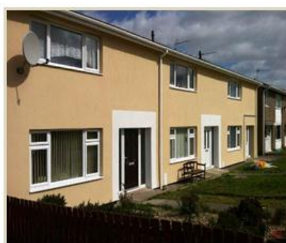
Radburn Estate , on completion
