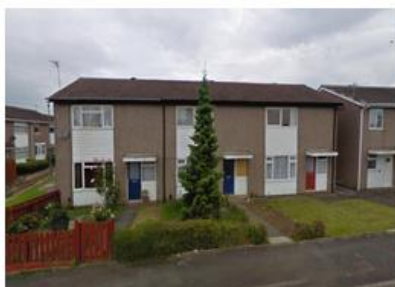
Radburn Estate , before works
