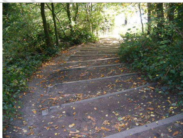
P4.5. Existing stepped access to the river
